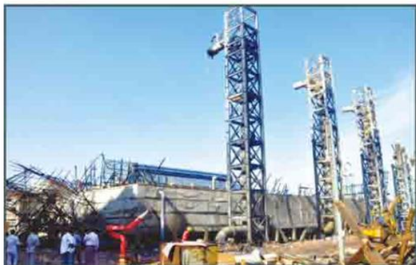
Figure 1. Cooling tower fire
