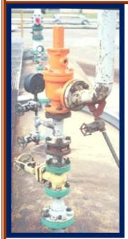
In the November 2012 *Beacon* many readers correctly identified one safety issue with the relief valve in the picture at left – potentially closing a block valve, isolating the relief valve so it cannot provide protection against excess pressure. A second possible problem, a piping system which may cause the relief valve to chatter, was not identified by nearly as many people.
